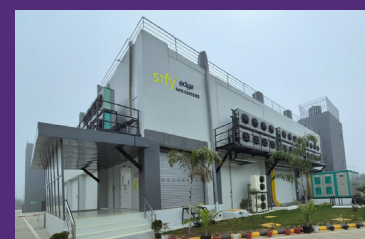
Lucknow 01 ⚡ 14 MW IT Capacity
