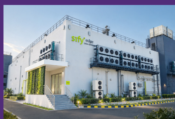
Chandigarh 01 ⚡ 4.8 MW IT Capacity
